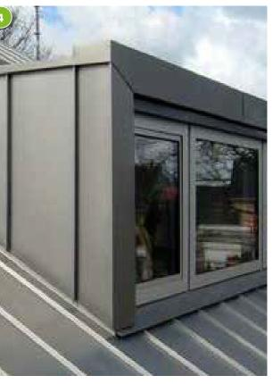
Powder coated (Grey zinc colour) standing seam pressed metal panel finish to box dormer roof detailing.
